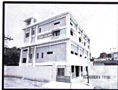
STP at Lawspet
