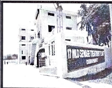
STP at Dubrayapet
