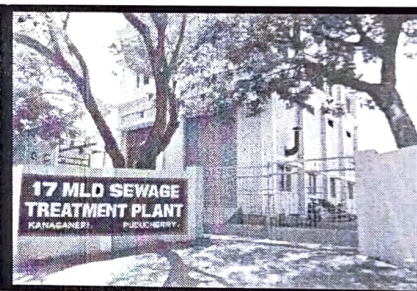
STP at Kanaganeri
